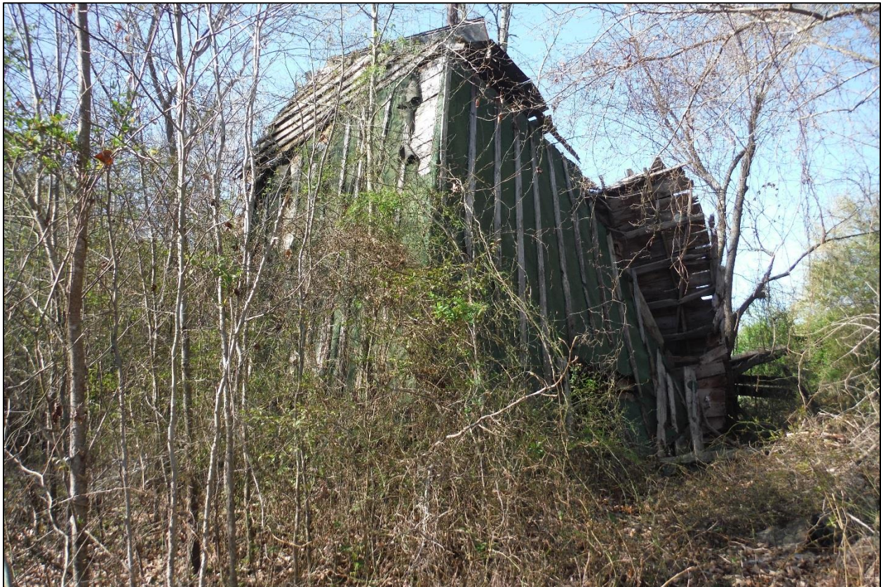
Figure 14. NS1555, Tobacco Barn 1, view to the southwest.
