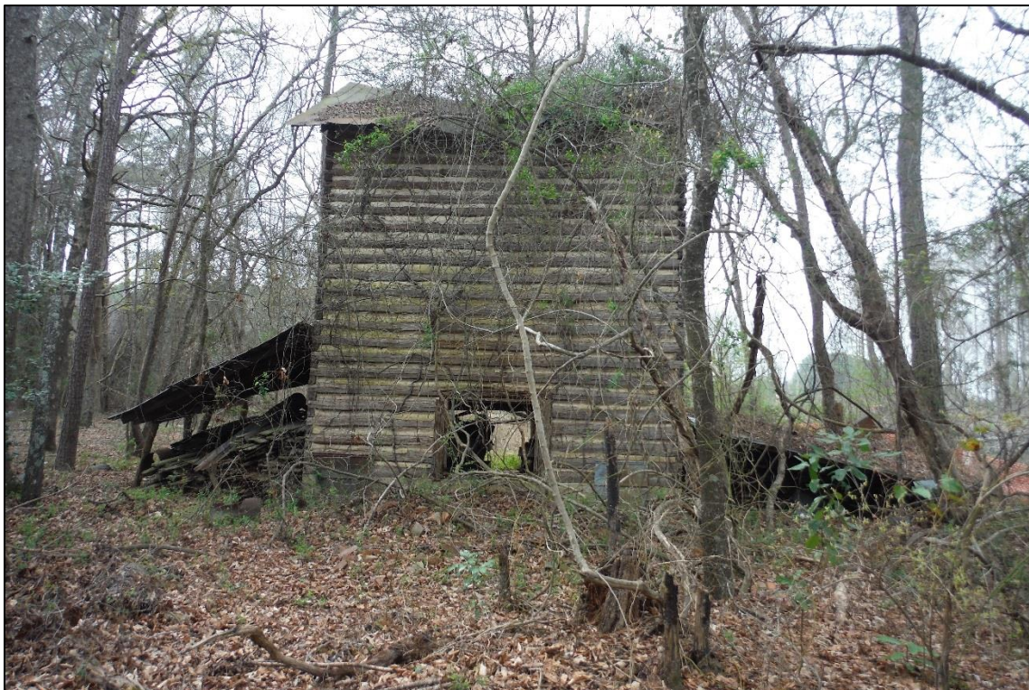
Figure 9. CD1480, east elevation, view to the west.
