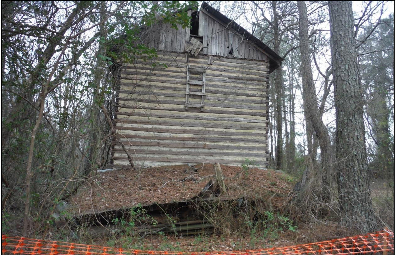
Figure 10. CD1480, north elevation, view to the south.
