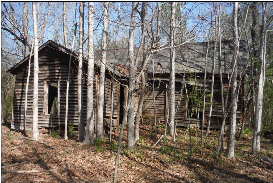
Figure 12. NS1555, view to the northwest.
