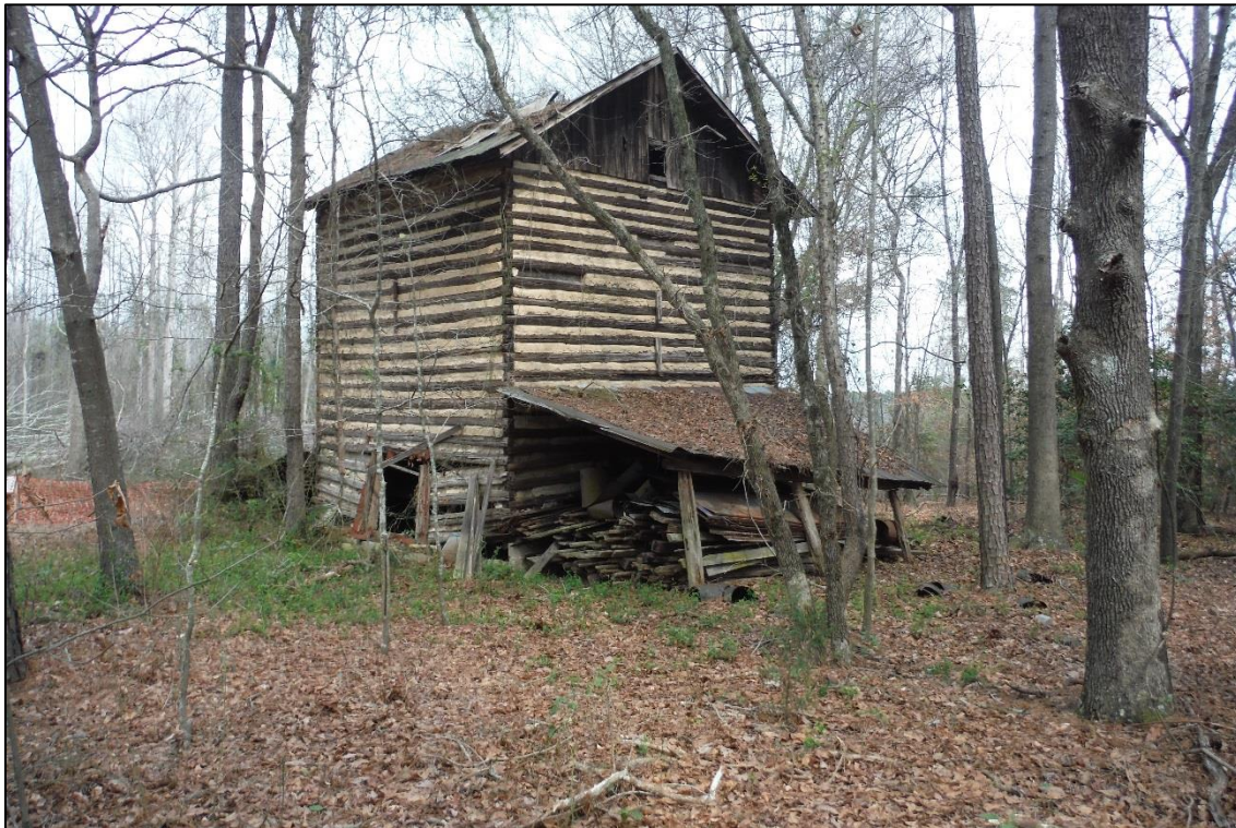
Figure 6. CD1480, south and west elevations, view to the northeast.
