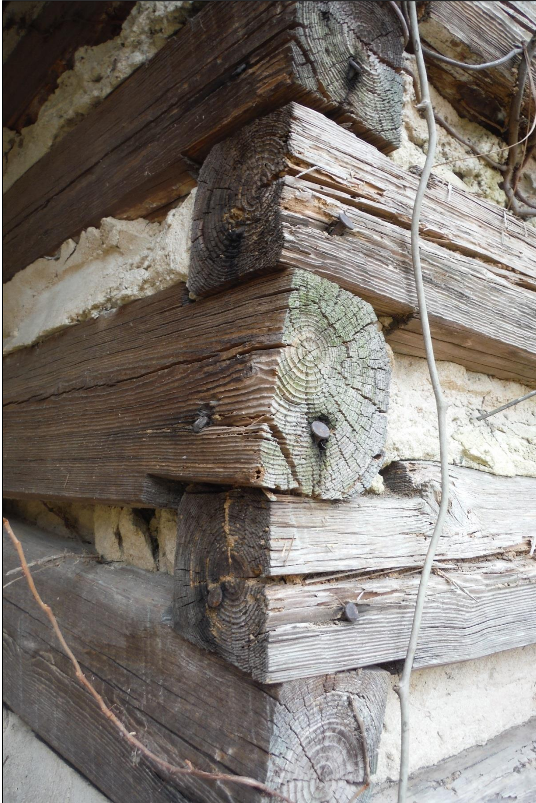
Figure 7. CD1480, southeast corner, view to the northwest.
